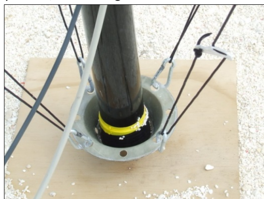
Fig. 24 Mast base of a VDA from 10m to 30m (Photo: Lagunaria DX Group)
